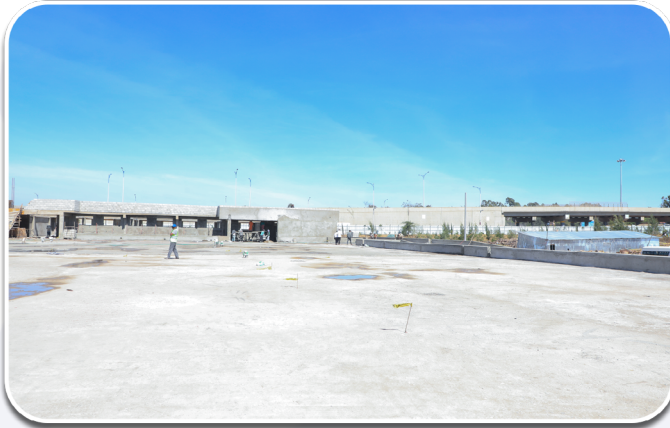
Excellence and Convention Centre Underway
