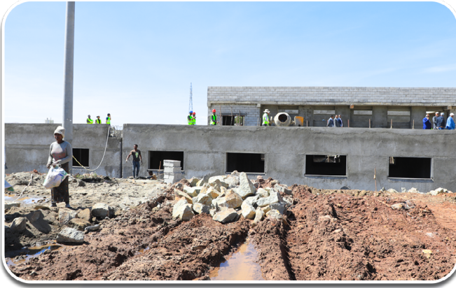
Excellence and Convention Centre Underway
